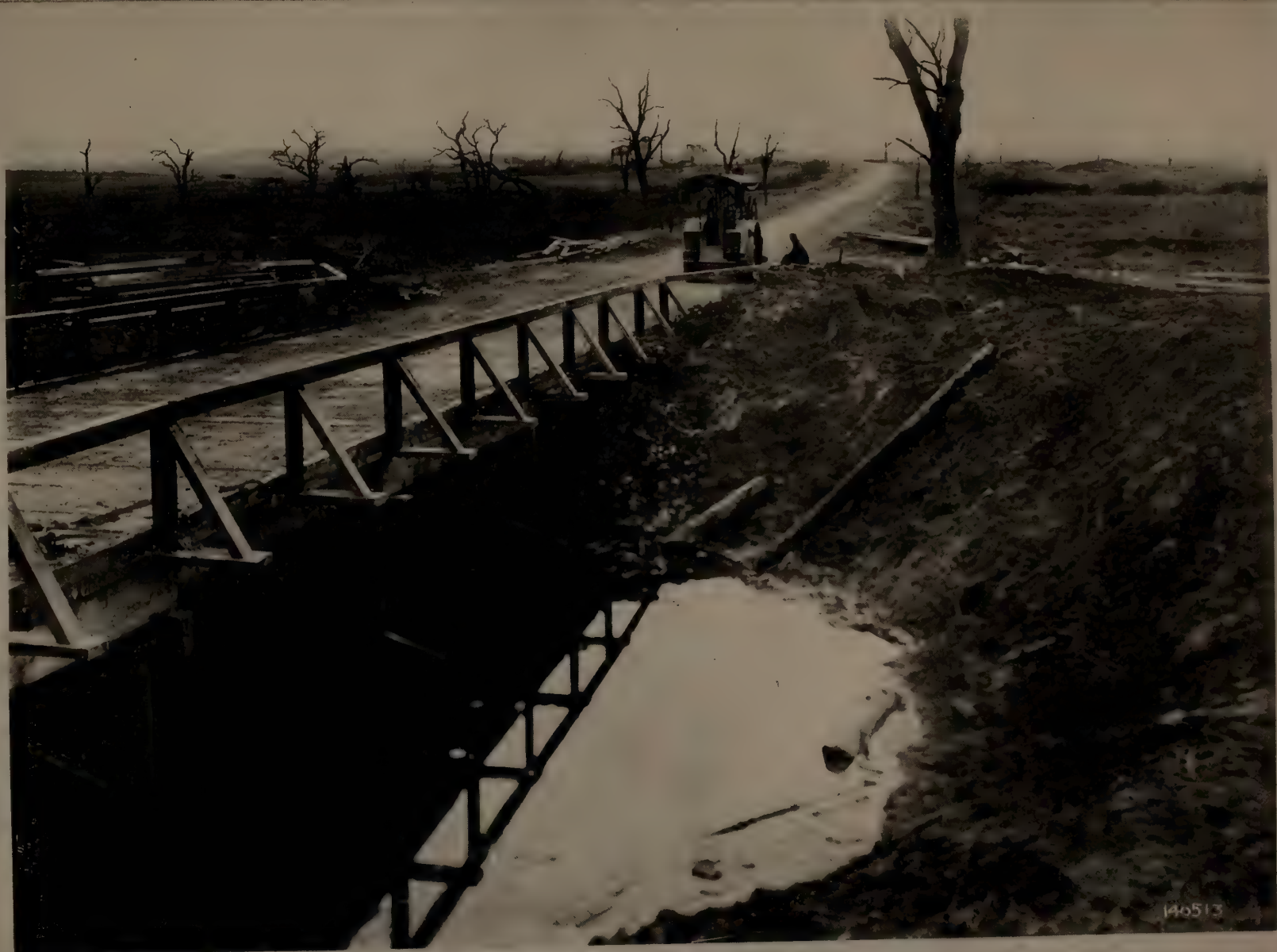
A Bridge across a Hole excavated by an Aerial Bomb.
